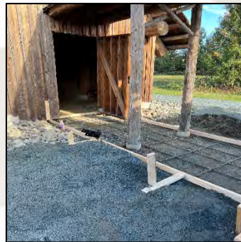
Forms for new Concrete walkway.
