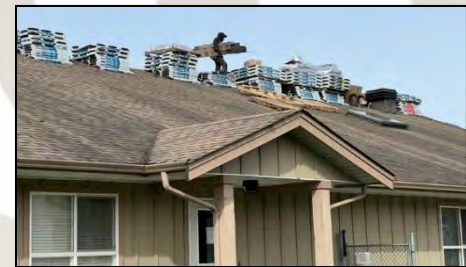
New roof install at the Á:Imélháwtwx Early Education Centre.
